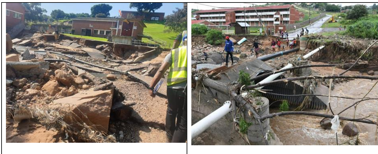
Figure 3.12 Infrastructure damage caused by Floods in KZN South Africa April 2022
